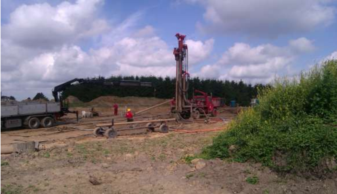
Fig. 6.4: Drilling of boreholes (2)
