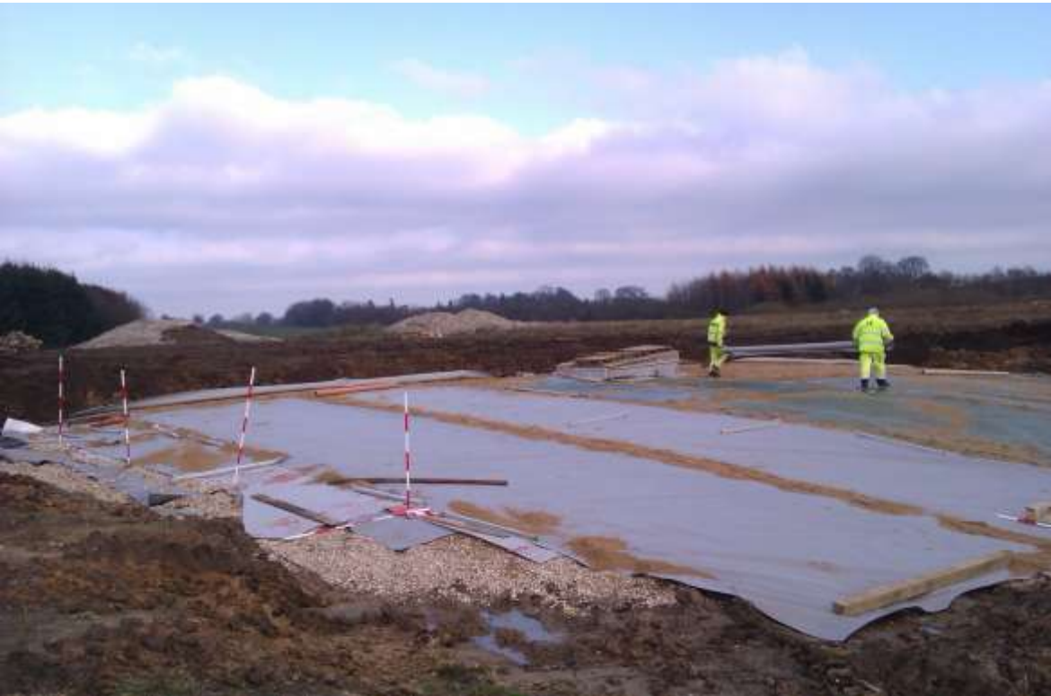
Fig. 6.8: Geo textile and semi permable roof foil placed upon cockle shells
