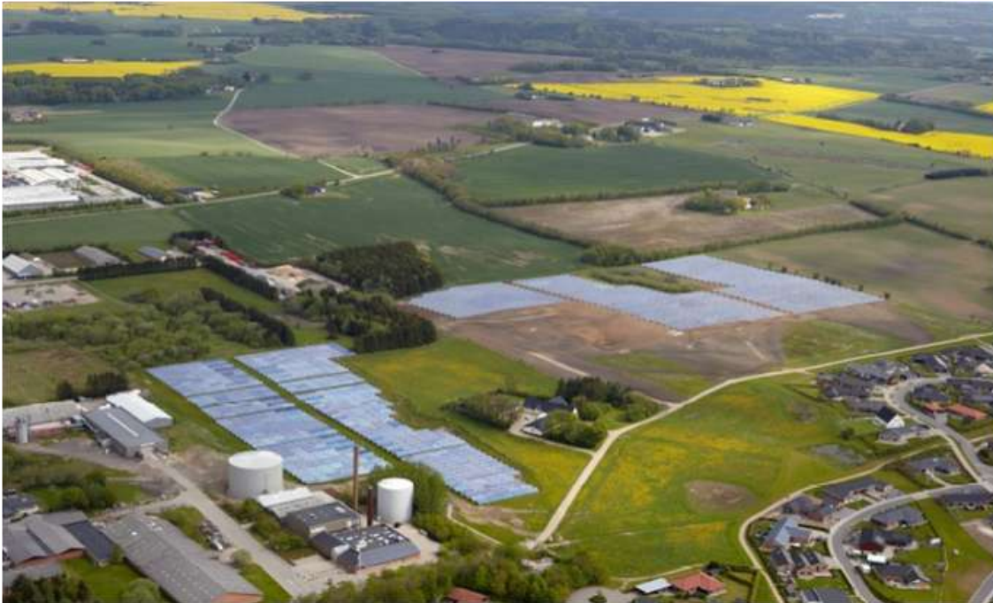
Fig. 6.13: Solar collectors and borehole storage implemented
