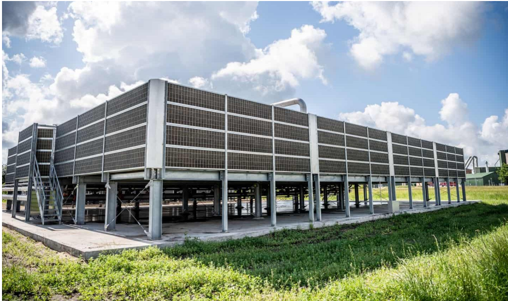
Figure 11. Evaporators with wall mount to reduce air recirculation at Karup Fjernvarme. (Credit: Morten Pedersen. https://viborg-folkeblad.dk/rundtomviborg/trods-gasprisernes-himmelflugt-lokalt-varmevaerk-styrer-flot-uden-om-prisstigninger#slide0 )
