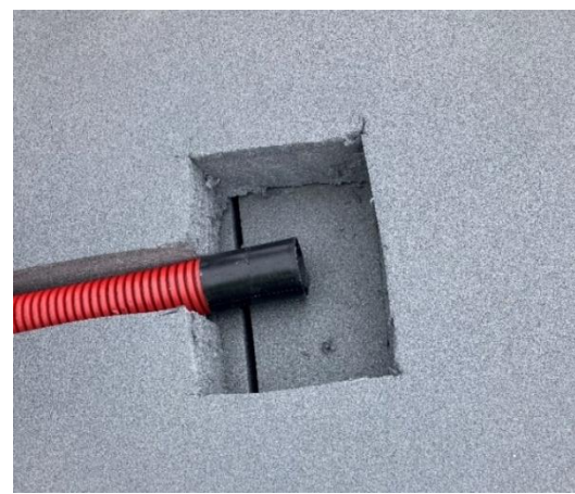
Cut-out in insulation for Hygro-Smart humidity sensor HS3
