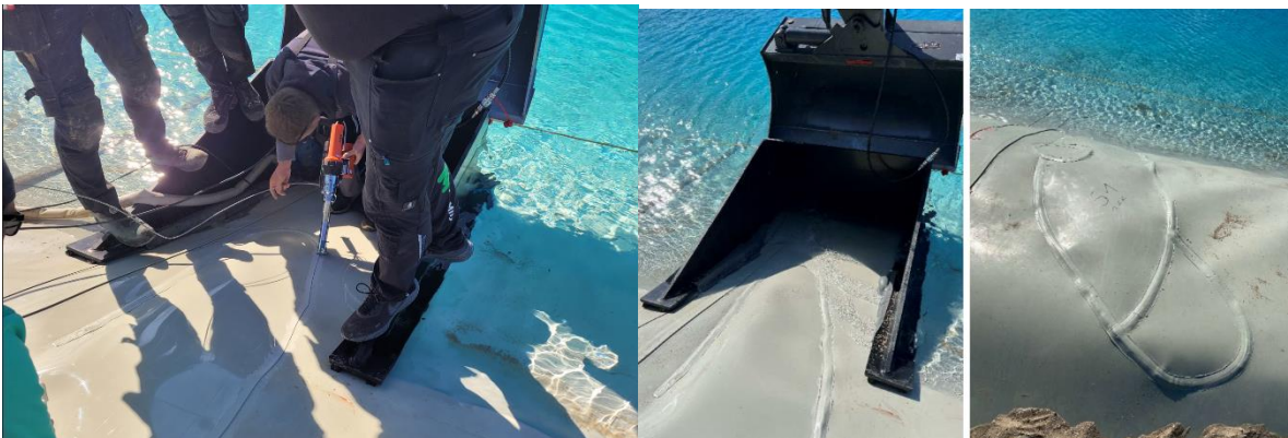
Figure 19: Repairing a crack using a caisson.
